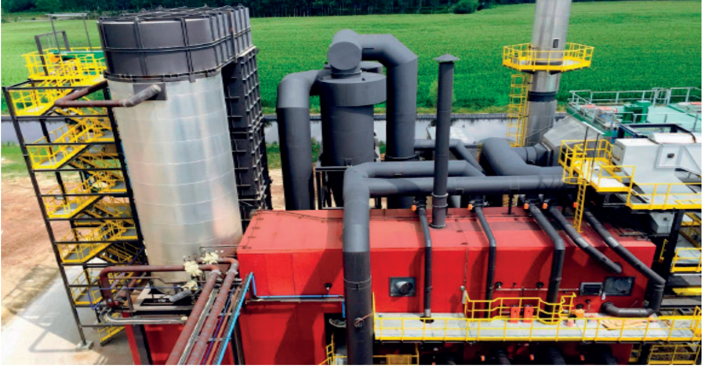
Biomass combustion plant with vertical adiabatic chamber – 12 MW - France
